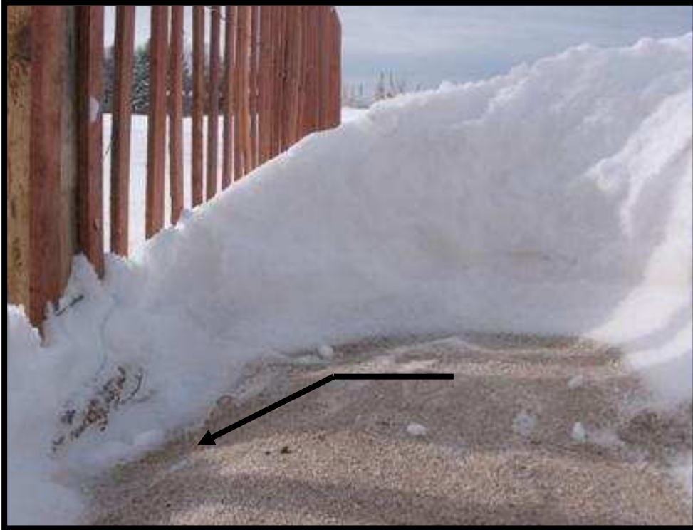
Figure 13: Sand build-up as a result of snow fence
