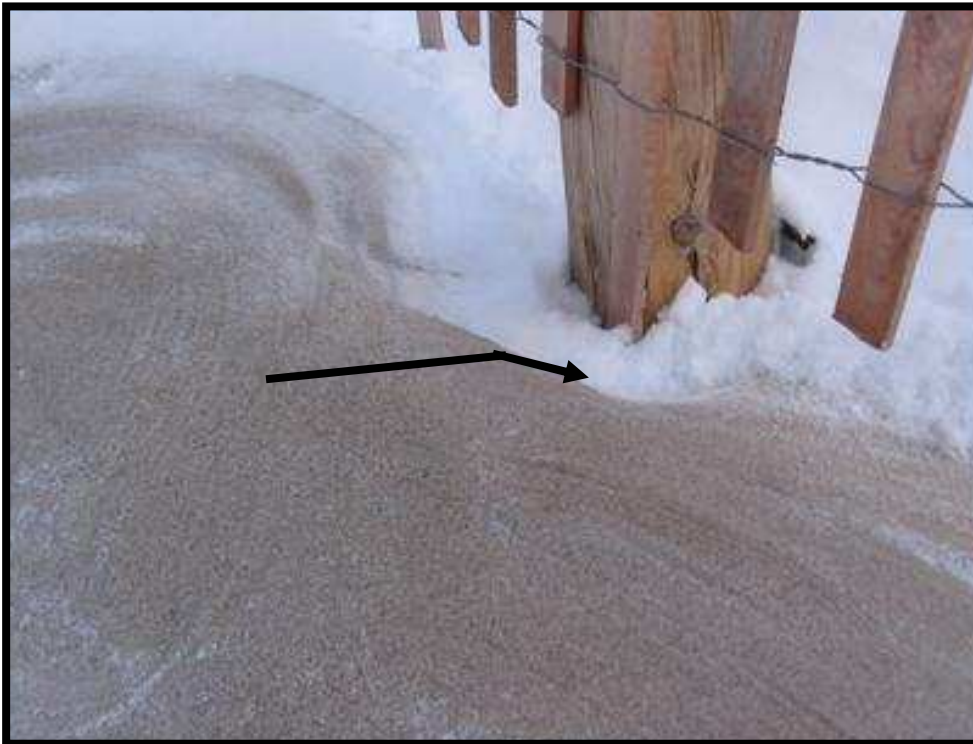
Figure 14: Sand build-up as a result of snow fence
